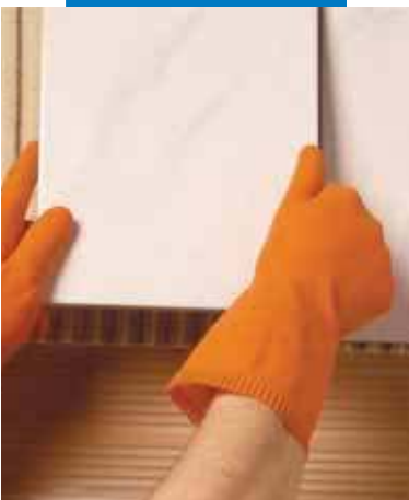
Fixing ceramic tile on wall
