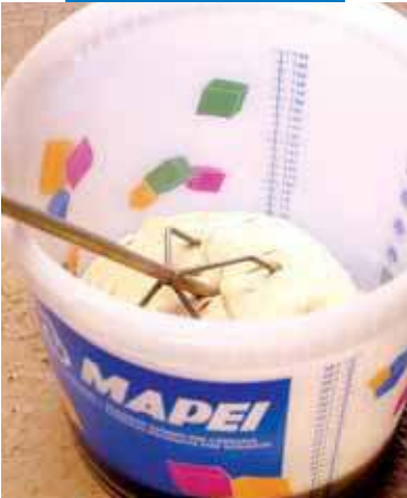
Mixing of Mapeset with a mechanical stirrer
